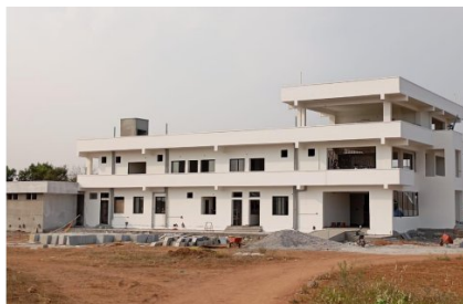
The new purpose-built Nireekshana Clinic building, currently an empty shell
